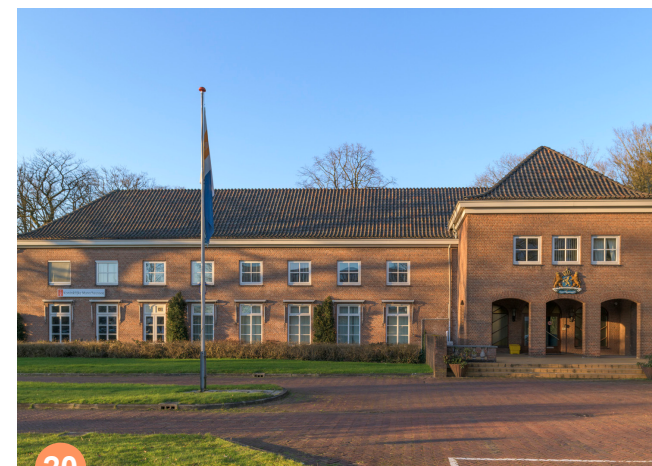
20 Royal Military Police Barracks (1956) Veldmaarschalk Montgomeryweg 2/Banningstraat, Soesterberg Architect unknown to us
