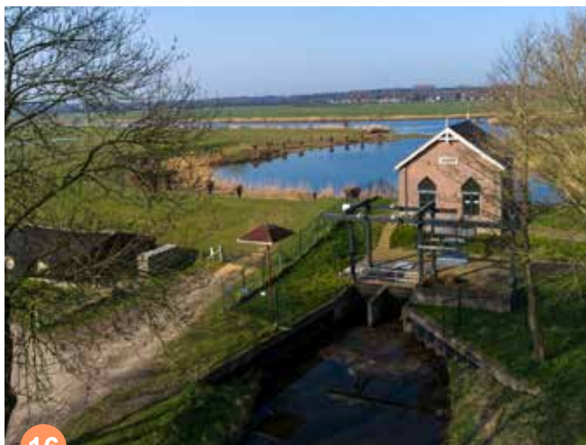
16 Zeldert pumping station (1896)
